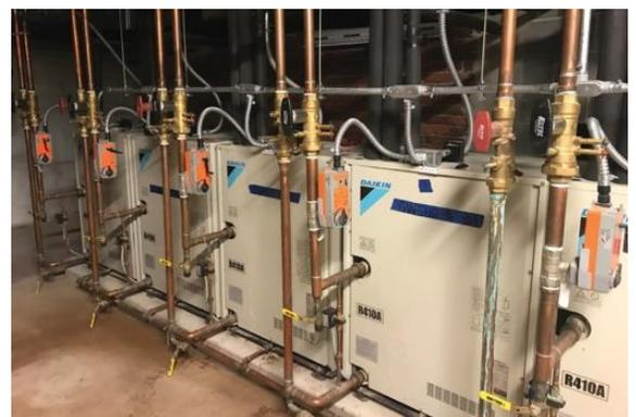
Havtech’s answer was to go ductless – an approach that minimizes penetrations into existing structures. Havtech and mechanical contractor Shapiro & Duncan, along with Global Engineering Solutions, proposed a Daikin water source VRV heat recovery system that allows customized zoning based on occupant demand.
