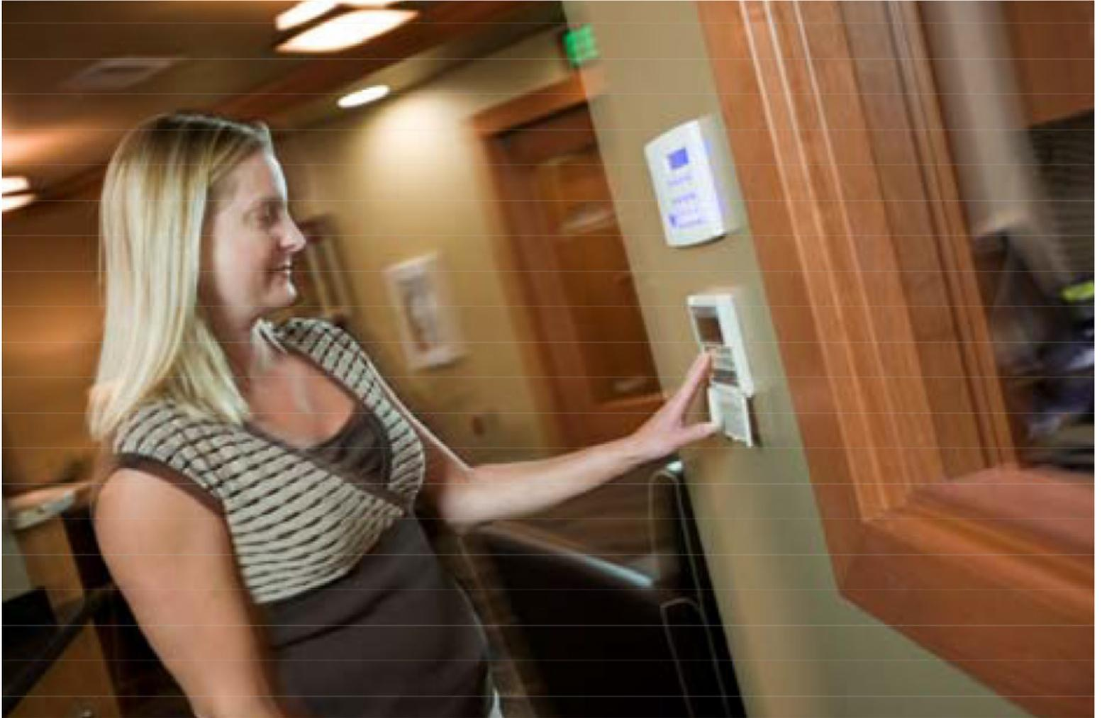
*The entire Daikin system, which stands completely alone from the rest of the building’s MEP systems, is controlled via Daikin remote sensors and 7-day programmable controllers.*
