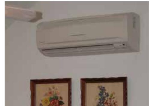
Aslan proposed using three 2-ton multi-split Daikin MXS heat pump systems, a simpler and more cost-effective multi-zone solution that fit the mansion perfectly. These replaced the two ailing 5-ton single split systems for a 40% reduction in tonnage that would take full advantage of building diversity and translate into good energy savings.
