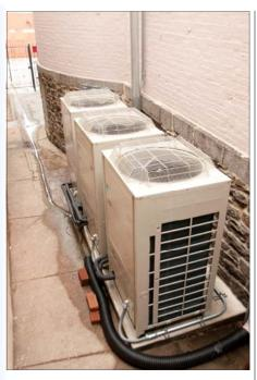
Daikin RXYQ outdoor condensing units at the rear of the synagogue which supply a total of 28 tons of capacity.
